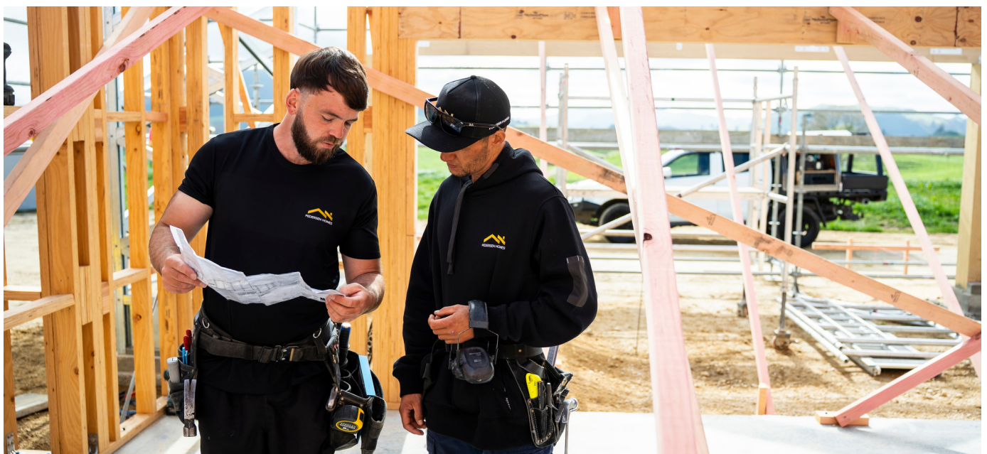
ON SITE, REVIEWING THE BUILD
